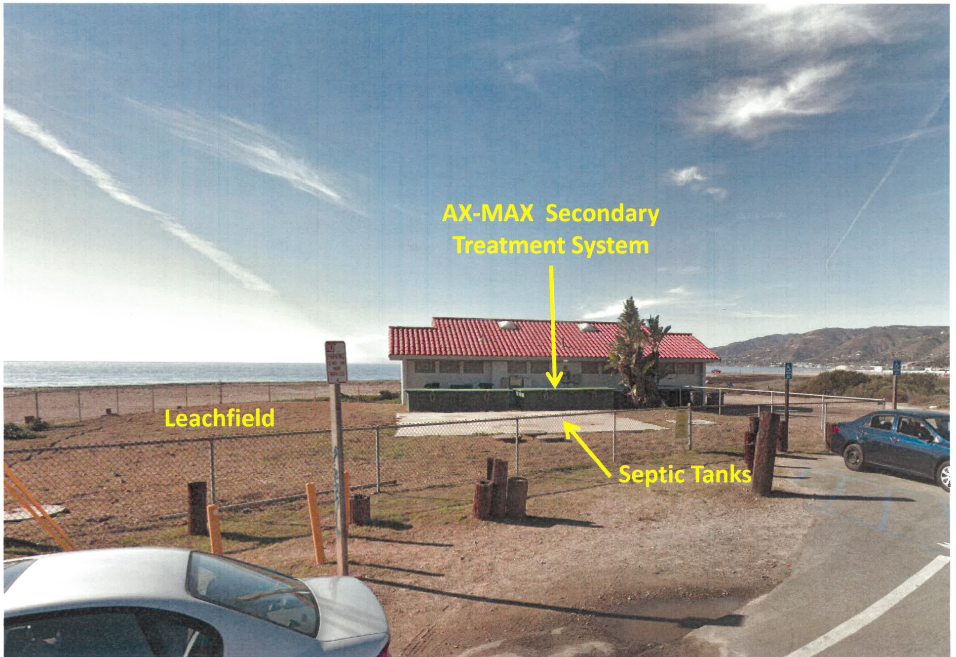
Zuma Beach Restroom Wastewater System
