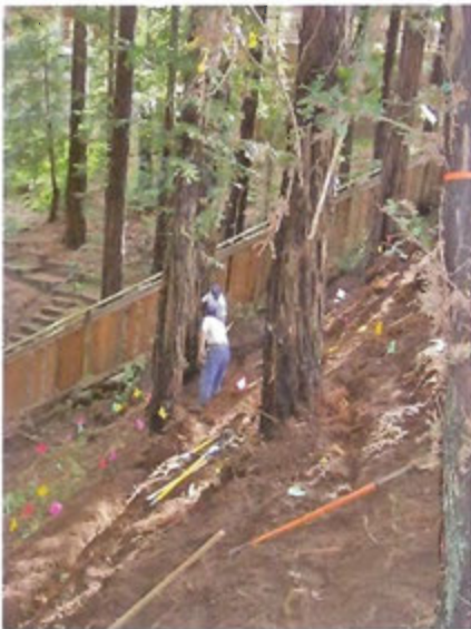
A steep slope installation in California — 65% slope.
