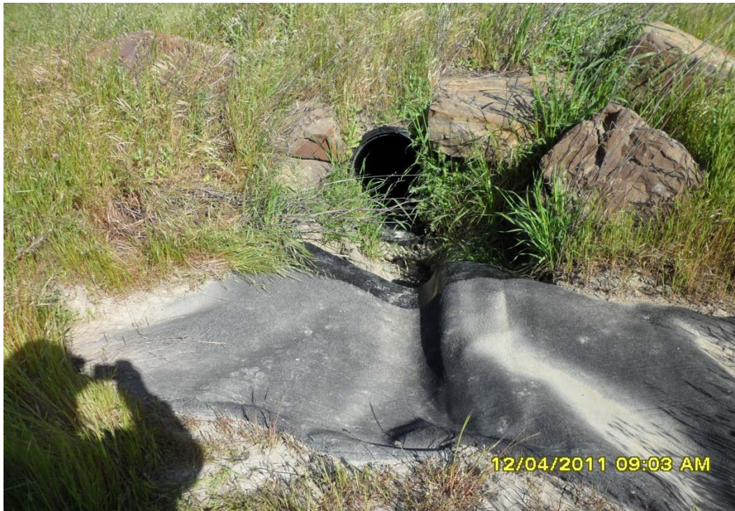
#3. Drainage pipe on the terraced slope adjacent to RAC/MRF site with tracks of raccoon.
