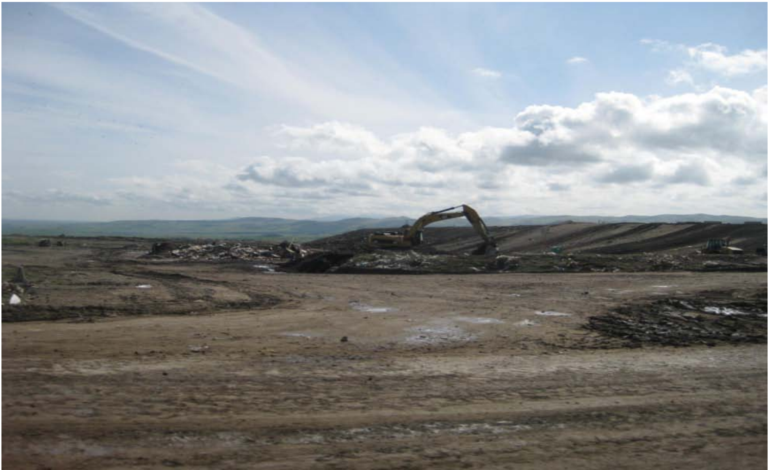
View #8- Active landfill area, facing east from northeastern portion of proposed organics management area.
